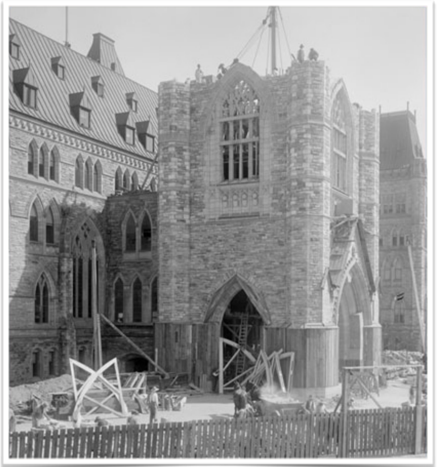
Peace Tower Under Construction in 1921
