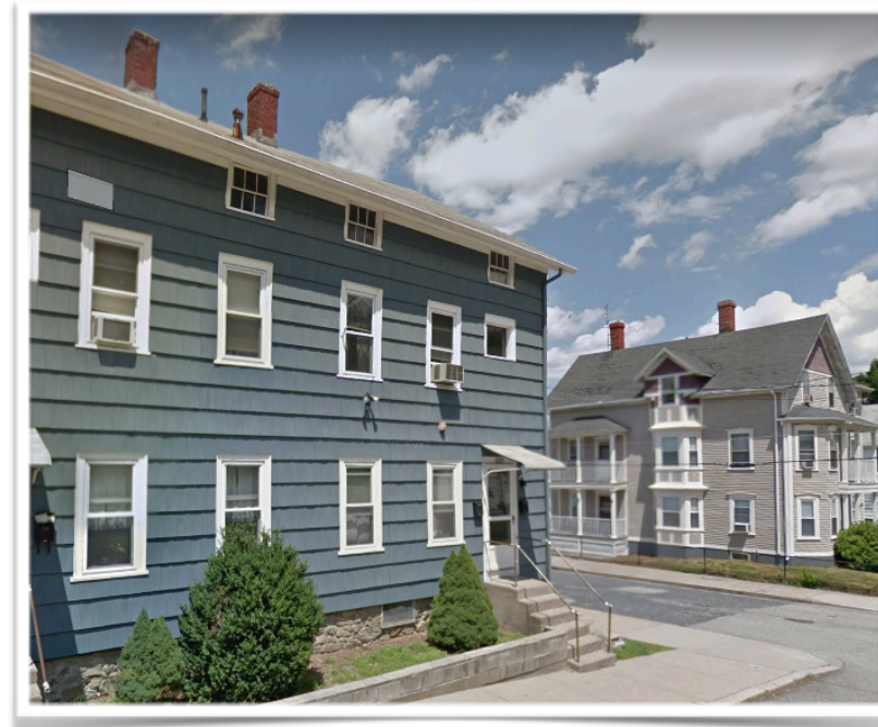
222 & 244 Paradis Avenue, Woonsocket, RI Photo from Google Maps 2022
