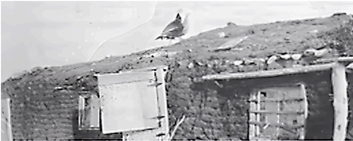
A sod barn ( Ecurie en terre ) on a homestead in the Lampman area, 1910 Poet's Corner
