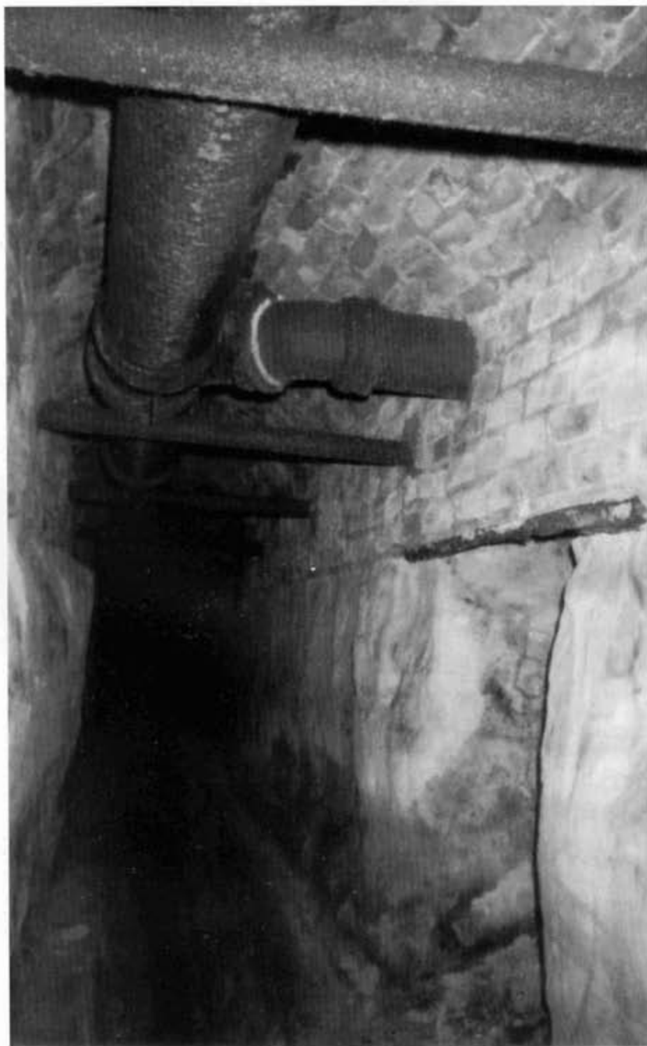
The Omaha sewer tunnel today. This photo by the author shows the Fountain Cave plumbing system. Strother's pipe runs along the ceiling. This sandrock tunnel was given a brick arch at places where it grazed the overlying tumblerock layer. The opening along the right wall leads to a sinkhole under the former Machine Shop. Initially, cavers thought that "sinkhole K" (point K on Strother's map) would provide a backdoor into Fountain Cave.
