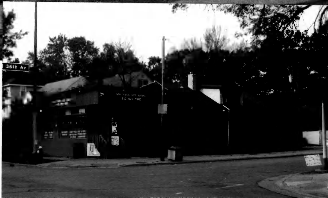
Views of 3559 Lyndale Avenue North Minneapolis MN (Collette store ca 1920)
