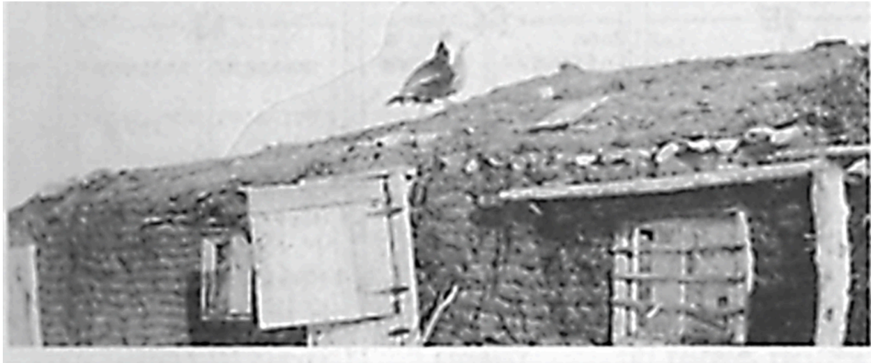
A sod barn ( Ecurie en terre ) on a homestead in the Lampman area, 1910 Poet's Corner
